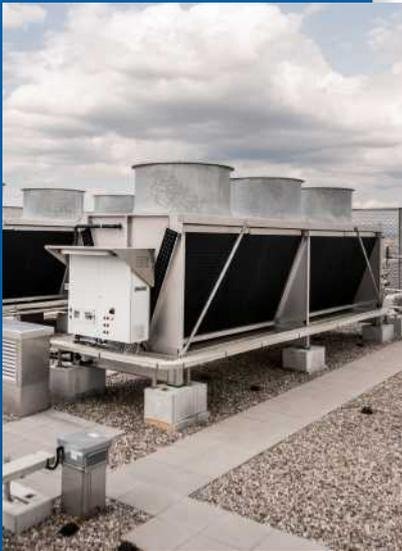
The JAEGGI *hybrid cooler* type *HTK* combines the function of an air-cooled dry cooler with a closed evaporative system. Depending on the required cooling capacity, free cooling is only supported additionally through evaporation of water from around 21 °C.
