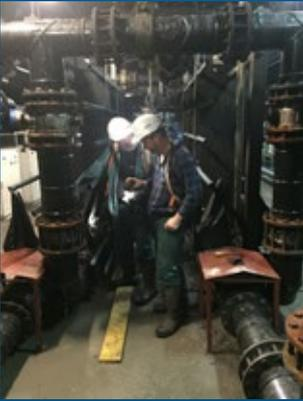
▲ The thermowave thermoline-Vario plate heat exchangers are designed to be especially corrosion resistant and can even withstand very unfavourable installation in the condensate without any restrictions.
