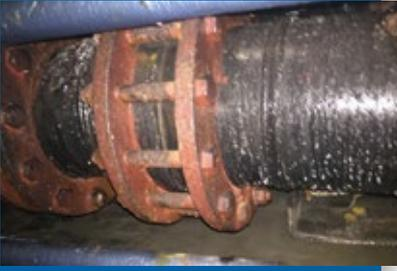
▲ The greatest adversary to technology installed underground is the highly corrosive atmosphere and high humidity and corresponding formation of condensation.
