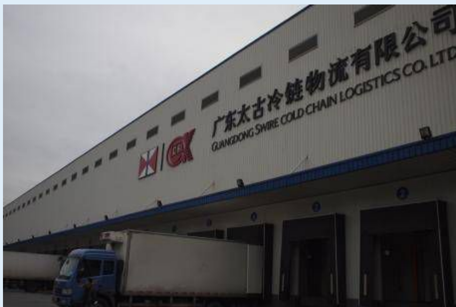
Guangdong Swire Cold Chain Logistics in Guangzhou, China
